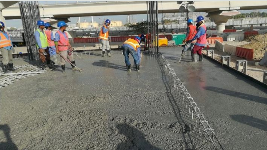
1. FOUNDATION AND BOTTOM SLAB WORK
